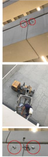
Two camera sites, covering ramps leading to First Floor of the Jamarat Complex. Two cameras were installed at each location, one to take images and the other for video.
